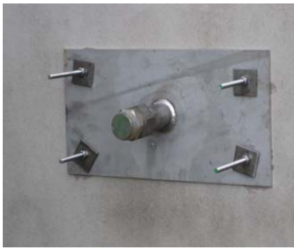
Figure 7. Lance bolted to the wall of house 3
